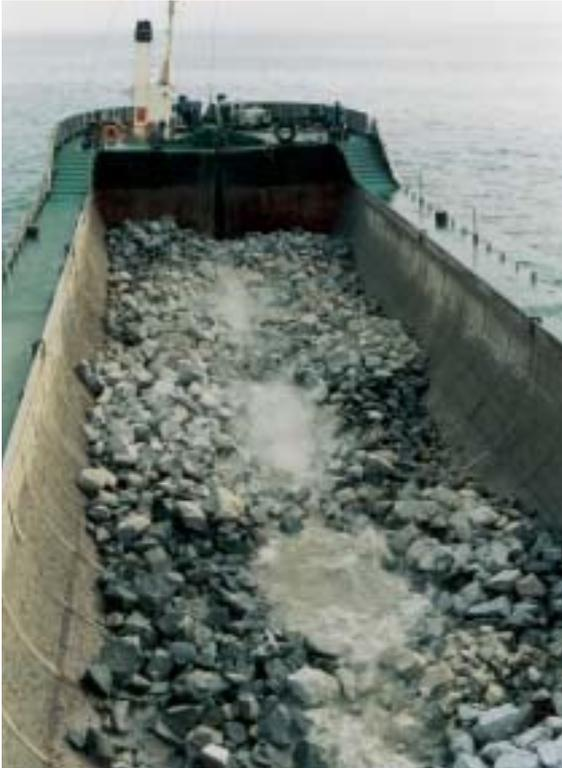
Figure 7. Installation of rockbund at Urmston Road by means of the 2000 m<sup>3</sup> self-propelled splitbarge Verrazzano.
