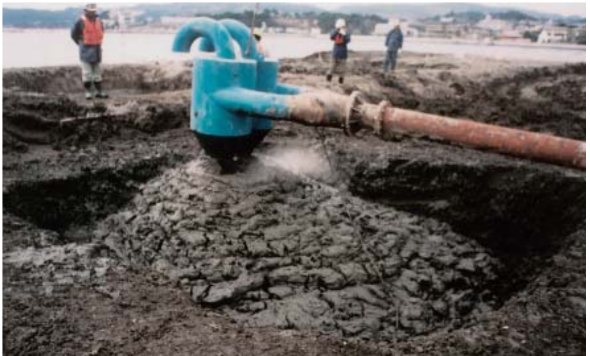
Figure 16. Discharge of solidifier and mud mixture.
