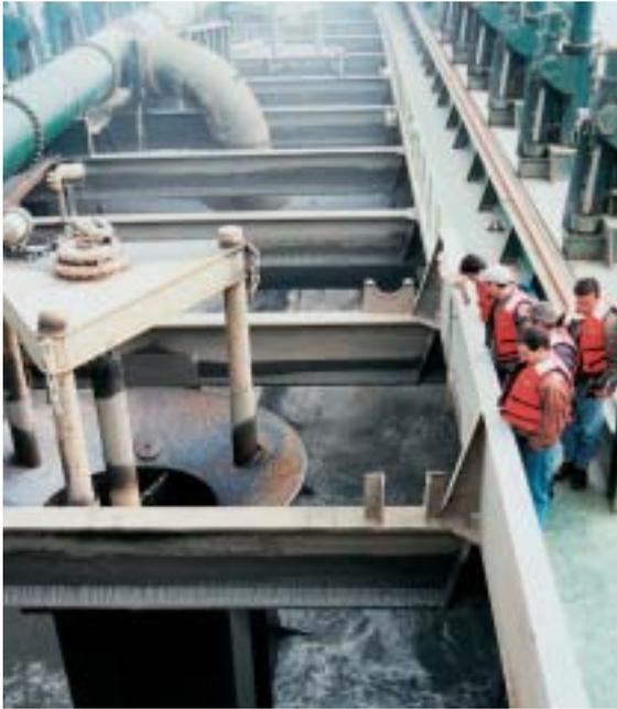
Figure 1. The hopper loading process seen here is similar to the process that takes place in sedimentation tanks of a water treatment plant.
