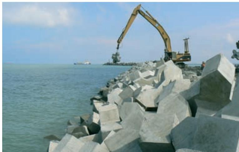
Figure 15. Xbloc® placement with the crane.
