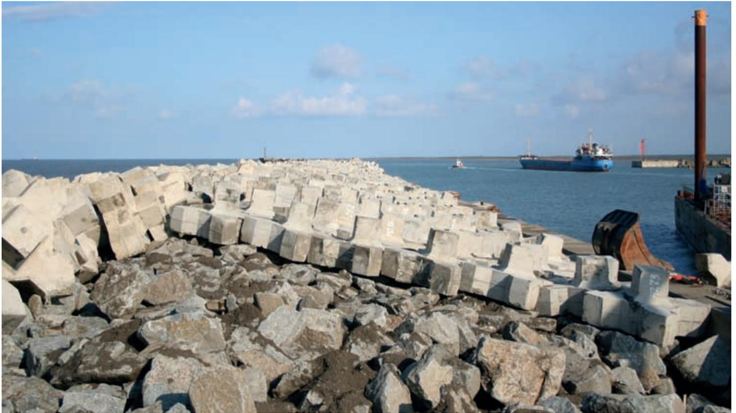
Figure 3. Xbase® layer on the crest of the breakwater.
