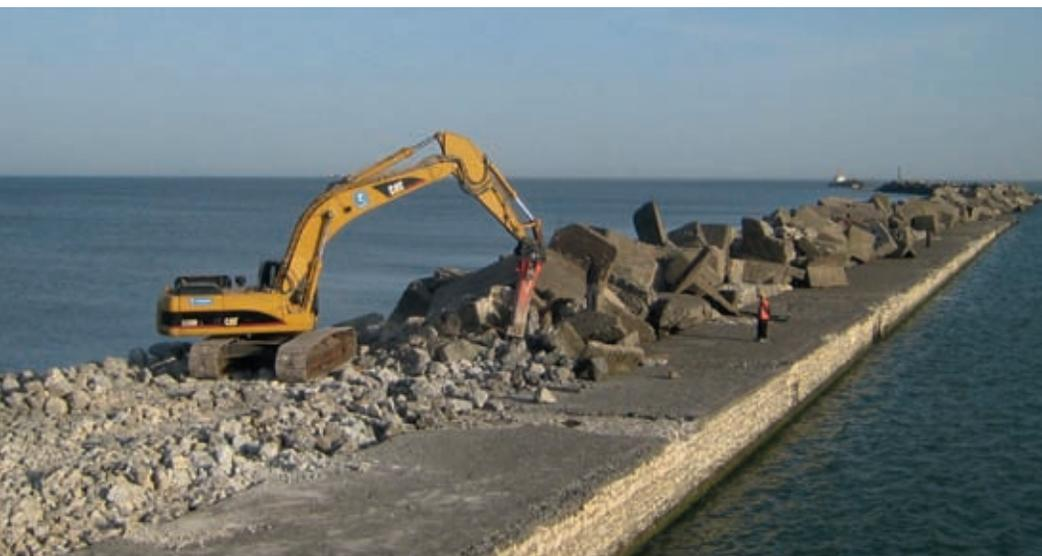
Figure 13. Destruction of the old blocks in a controlled manner using hydraulic hammers.
