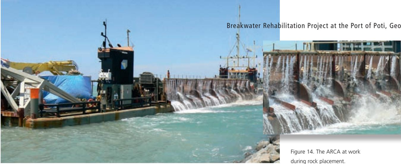
Figure 14. The ARCA at work during rock placement.
