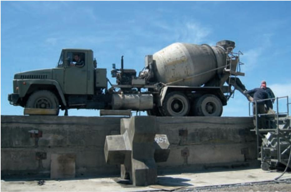
Figure 10. Xblocs® being poured from concrete mixing truck.
