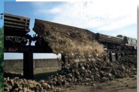
Figure 9. Loading (left) and unloading (right) of rock from the railway transport wagons.
