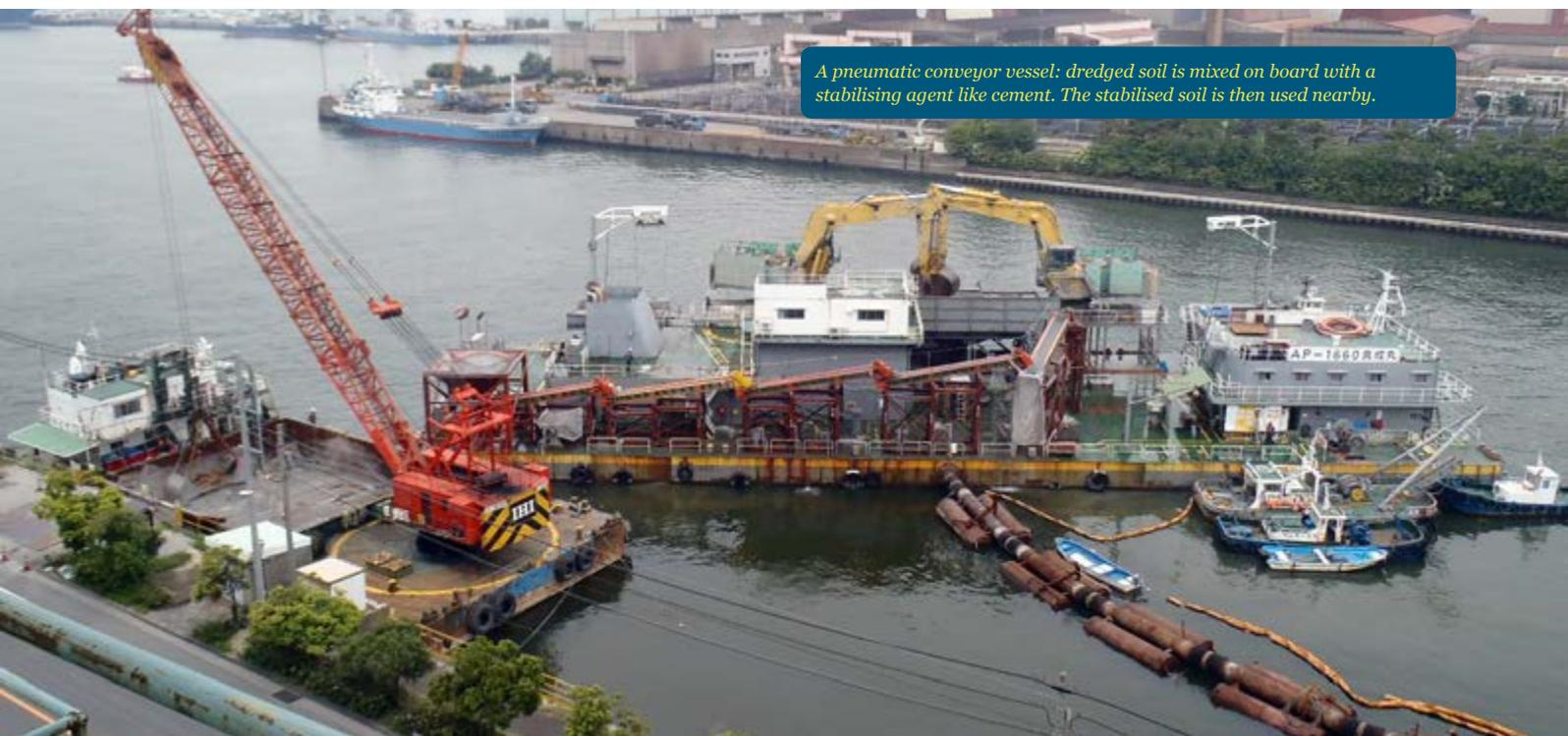
*A pneumatic conveyor vessel: dredged soil is mixed on board with a stabilising agent like cement. The stabilised soil is then used nearby.*
