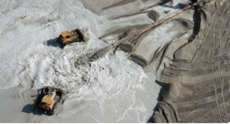
Left, compaction is being carried out with bulldozers in front of the discharge pipe. Right, HEIC is done by impact rollers equipped with modules weighing upwards of 8 tonnes pulled over the new land by tractors.
