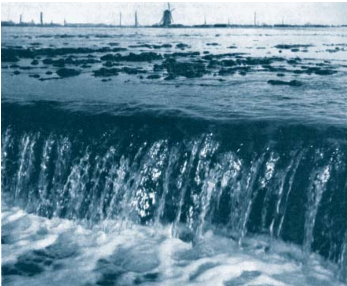
Figure 4. In some cases the streaming water through the breaches in the dikes caused deep gullies and waterfalls to form, which were difficult to close.
