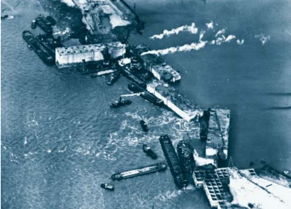
Figure 5. Caissons being used to close the gap at Ouwerkerk. The extent of the repair work was enormous.
