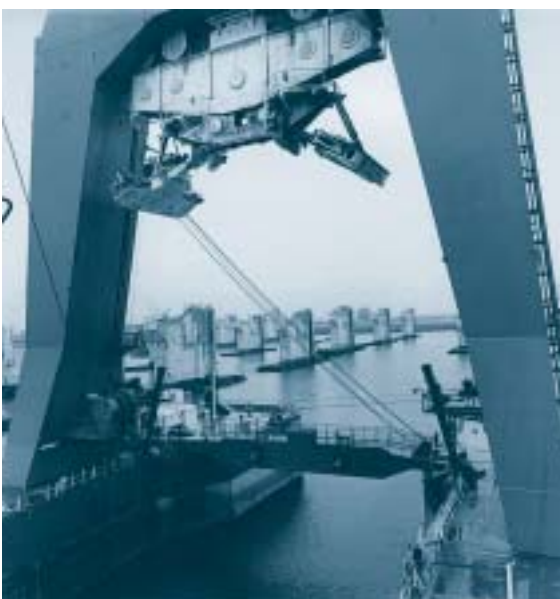
Figure 8. Concrete piers at the Oosterschelde works.
