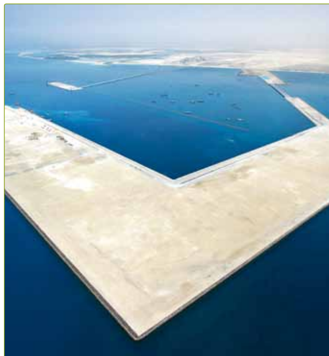
Land reclamation platform for the new Khalifa port, Abu Dhabi
