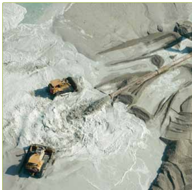
Soil compaction using bulldozers
