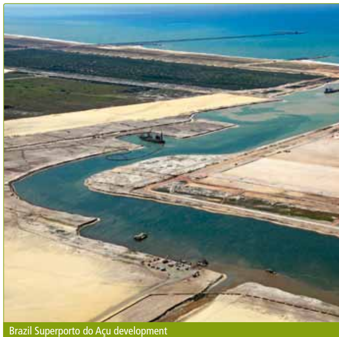
Trailer rainbowing hydraulic fill
