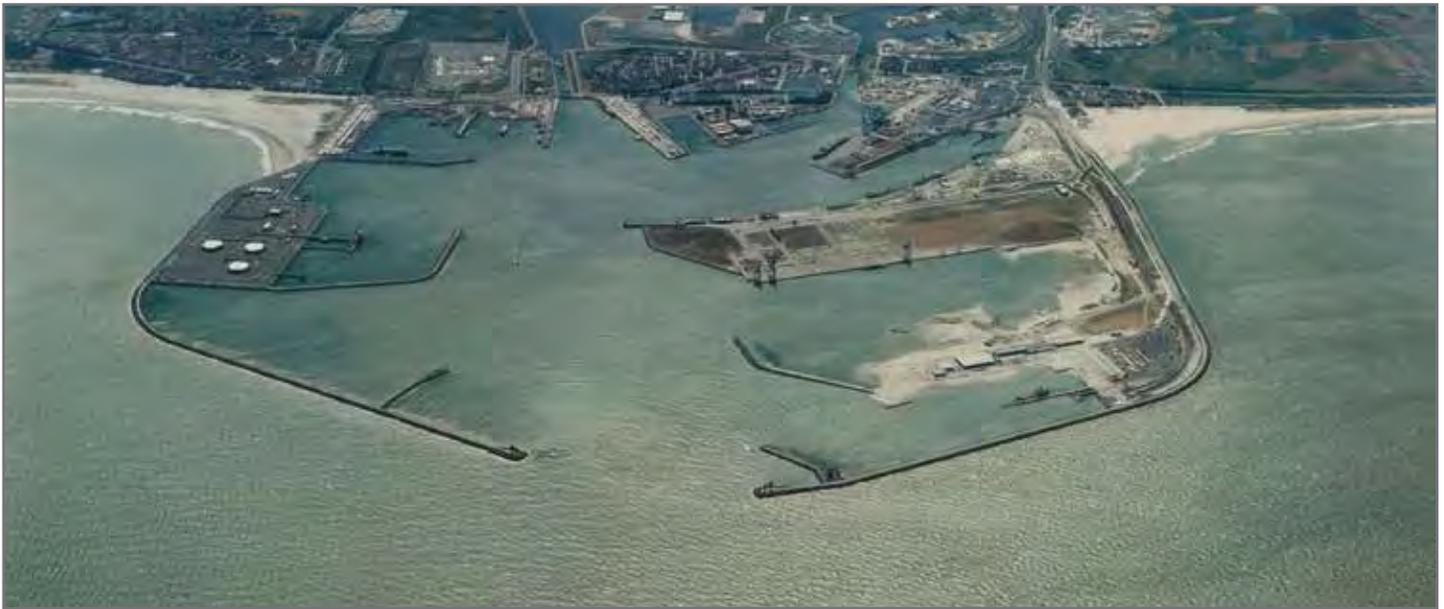
*Beginning in 1977, the Port of Zeebrugge, Belgium expansion began, adding breakwaters and terminals, and deepening the port basin. More than 30 million cubic meters of material were dredged in the project, which was completed in 1999.*
