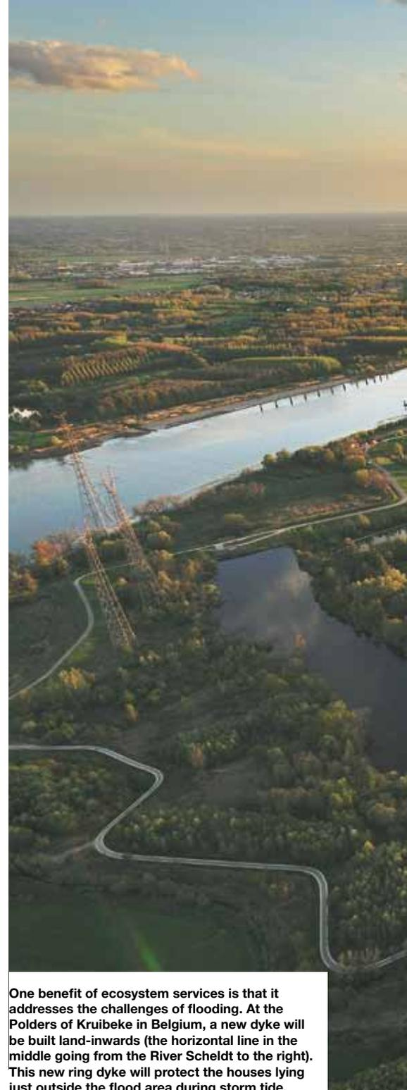
**One benefit of ecosystem services is that it addresses the challenges of flooding. At the Polders of Kruikeke in Belgium, a new dyke will be built land-inwards (the horizontal line in the middle going from the River Scheldt to the right). This new ring dyke will protect the houses lying just outside the flood area during storm tide.**
