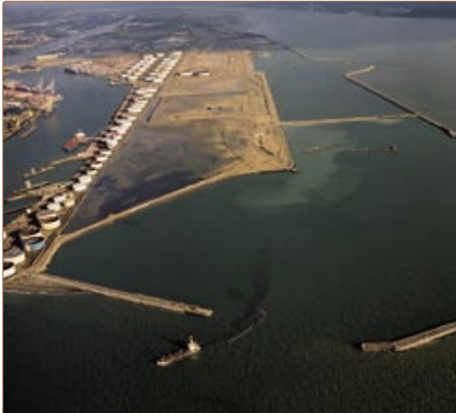
Aerial view of the work at the Port 2000 at Le Havre: Expansion of the port will guarantee that the French harbour will be able to accommodate increasingly larger container ships as well as an increase in shipping traffic.
